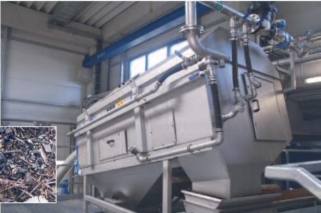
ROTAMAT® Wash Drum for washout and separation of all coarse material > 10 mm Grit classifying and washing
